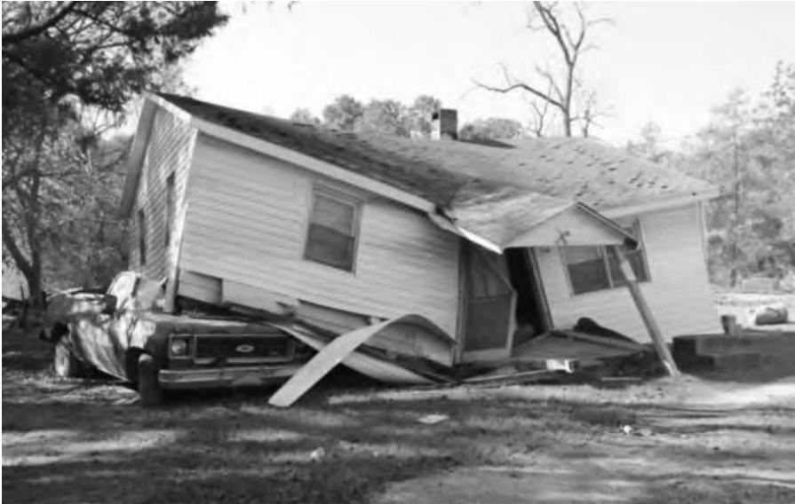
Figure 122 Princeville, NC, November 8, 1999. The September floodwaters brought by the rains from Hurricanes Dennis and Floyd left much devastation. The historic town of Princeville, North Carolina was almost totally covered by floodwaters. Here is one of the many buildings that were not strapped to their foundations. It apparently floated atop the family truck during the flooding—both a total loss.
