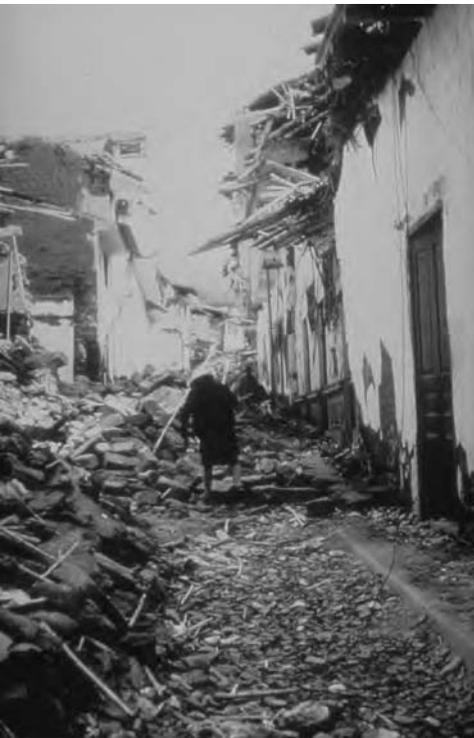
Figures 85 and 86 Photo (top) shows a city street in Huaraz before the earthquake. This adobe construction is typical of much of the housing that underwent complete collapse in the Andean townships. Photo (left) shows a city street in Huaraz after the earthquake.
