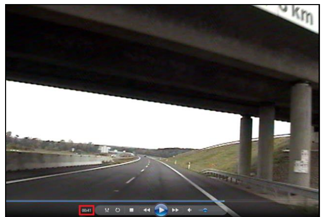
Fig. 7: Appearance of a bridge and its shadow at T=41s
