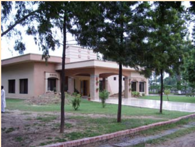
Ladies room constructed in 2005
